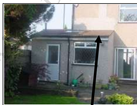
Shallow pitched roof to kitchen extension
