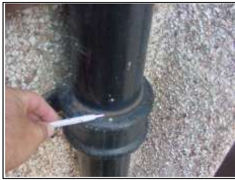
Minor rusting on soil and vent pipe that is expected on cast iron
