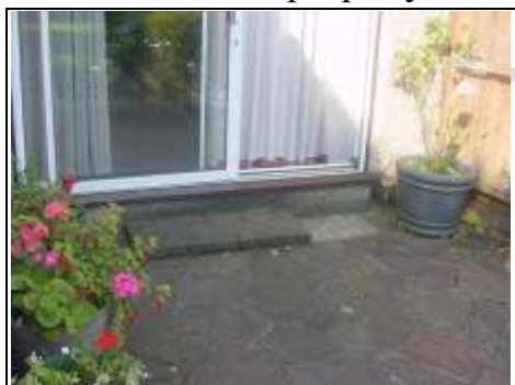
Patio doors with blocked air bricks
