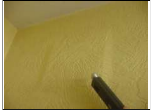
Internal air vent wallpapered over
