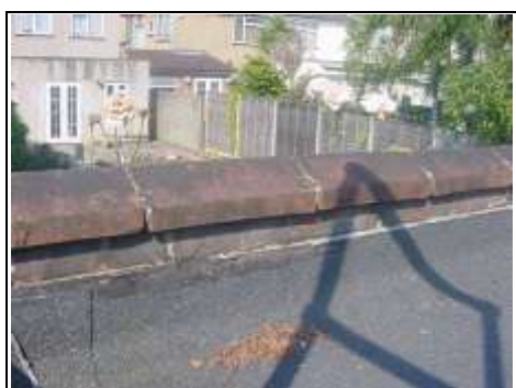
Parapet wall needs re-pointing
