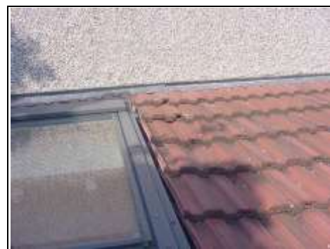
Shallow pitch of roof (remember to keep guttering around roof lights clear)
