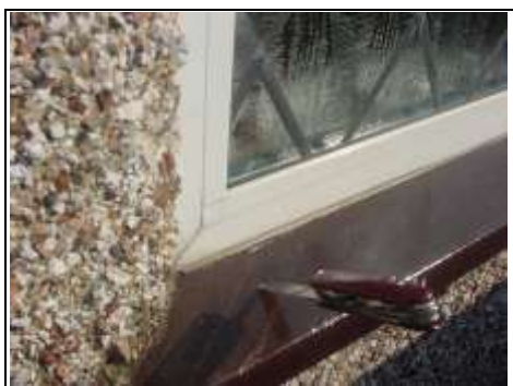
Testing the timber windows with a knife
