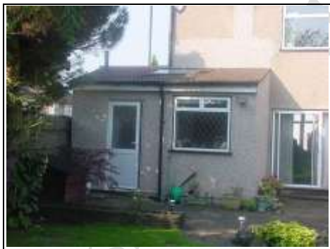
Shallow pitched roof to kitchen extension
