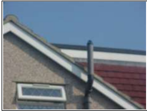
Soil and vent pipe
