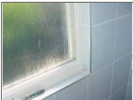
Thin walls in loft conversion (en-suite shower room)
