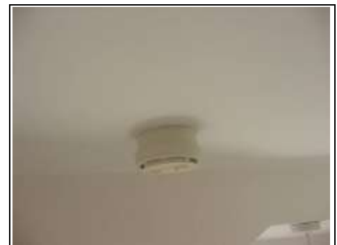
Hard wired smoke alarm
