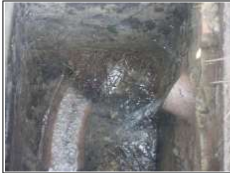
Drain (rear) with tree roots coming through
