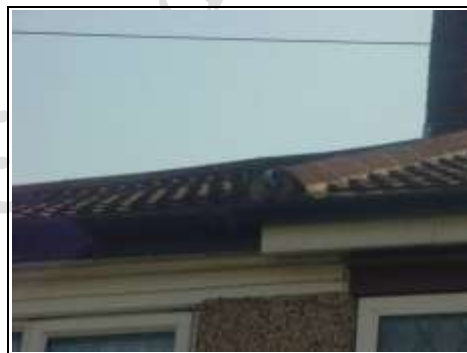
Hog backed tiles between the two roofs that indicate they were put on at different times.
