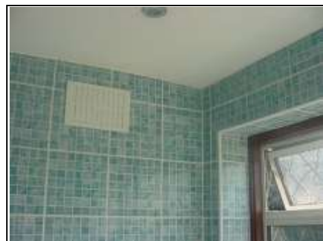
Large humidity controlled extract fan required in bathrooms and kitchen
