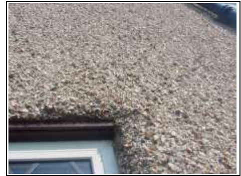
No drip detail over the window
