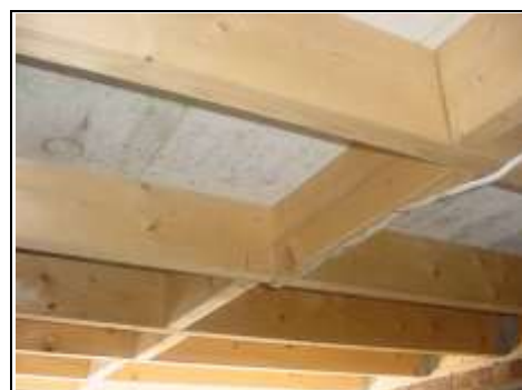
Mould indicates condensation is occurring
