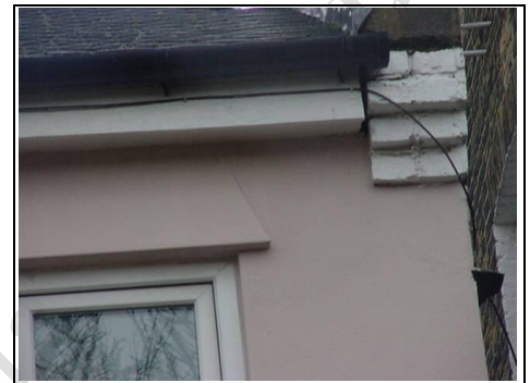
Drip details over the window on the render to the rear
