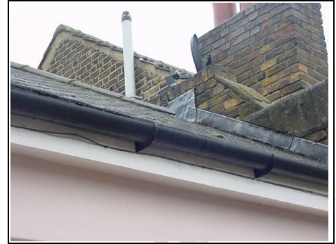
Soil and vent pipe
