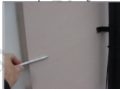
Old cracks that have been repaired previously
