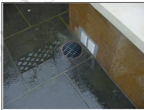
Airbrick acting as a gutter
