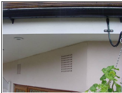
Crack at high level
