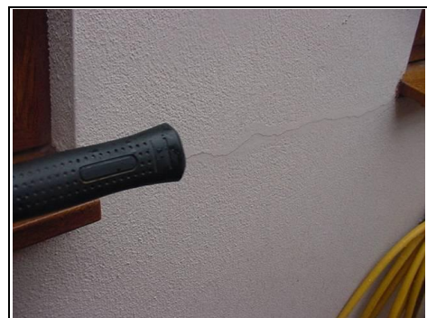
Cracking to the render
