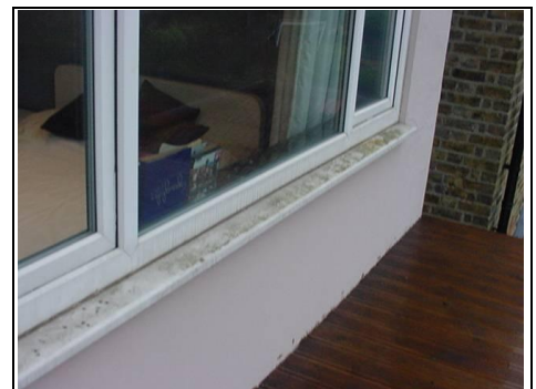
Wood decking covering the roof. Here we can see where the decking meets the main wall where there is no flashing
