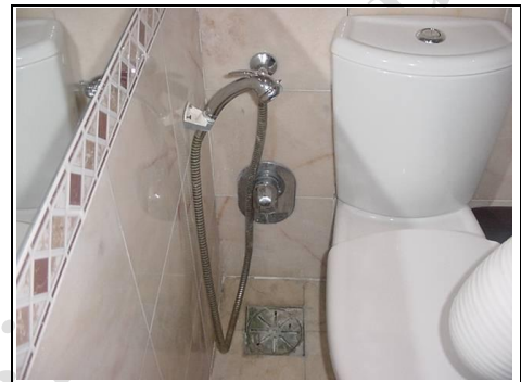
Washer unit in downstairs w.c. is leaking
