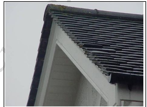
Tiles slightly displaced to the front
