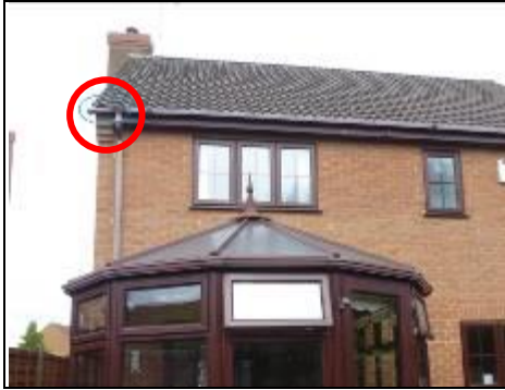
Rear right gutter dropping
