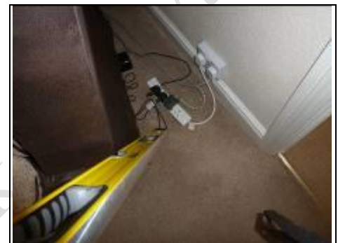
Additional socket points required
