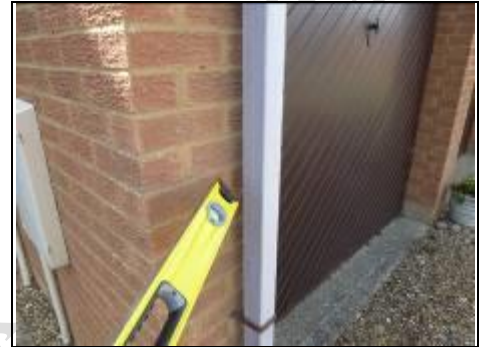
Faded plastic downpipe
