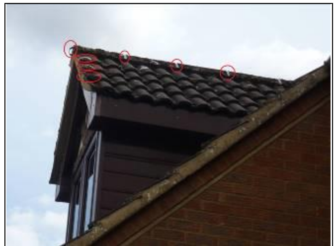
Dormer window has clips on tiles
