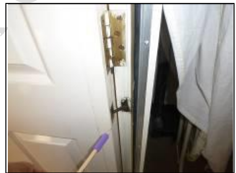
Internal door closer to garage
