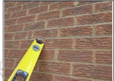
Stretcher bond brickwork
