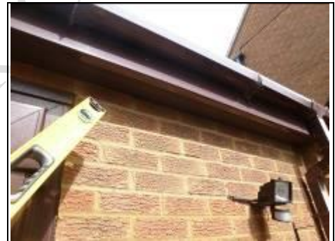
Vented soffit
