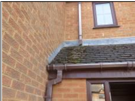
Leaking gutters and downpipes
