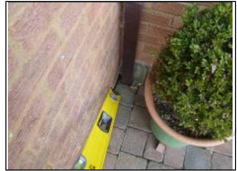
Downpipes feed directly into ground
