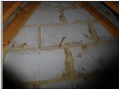
Horizontal crack
