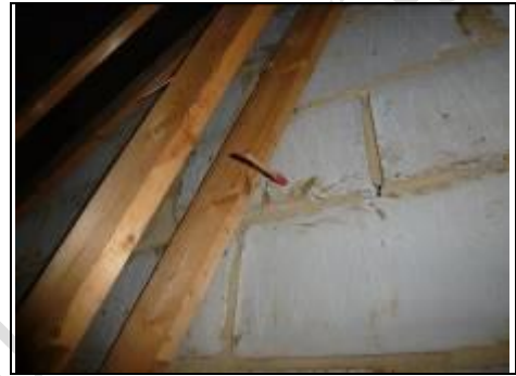
Raking crack
