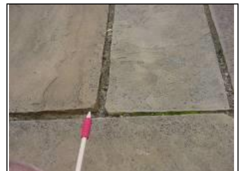
Paving slabs need levelling up
