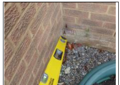
Airbrick to front right around chimney
