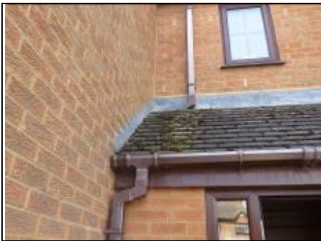
Leaking gutters and downpipes
