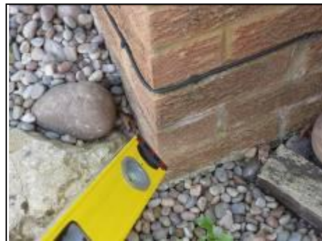
Water damage/efflorescence to base of brickwork
