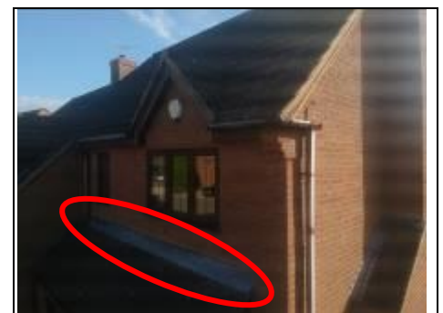
Cement mortar to lead flashing likely to come away
