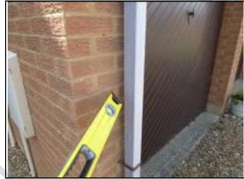
Faded plastic downpipe
