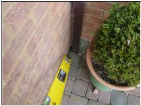
Downpipes feed directly into ground
