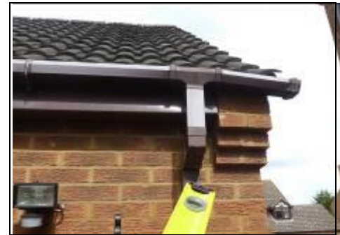
Unsupported gutter to rear left
