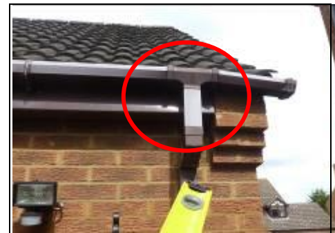
Unsupported gutter to rear left
