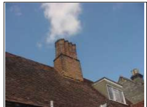
Rear left hand side chimney letting in light and dampness to property
