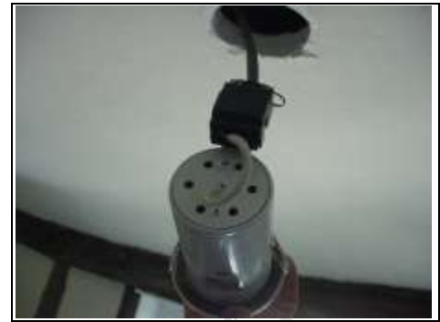
Light fitting giving heat directly into floor and roof space
