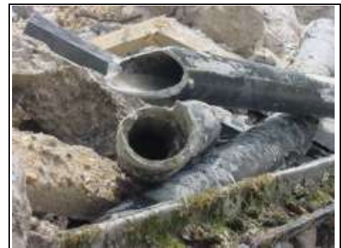
Asbestos pipes removed and not bagged for disposal
