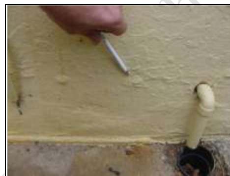
Old inserted damp proof course to right hand side main building
