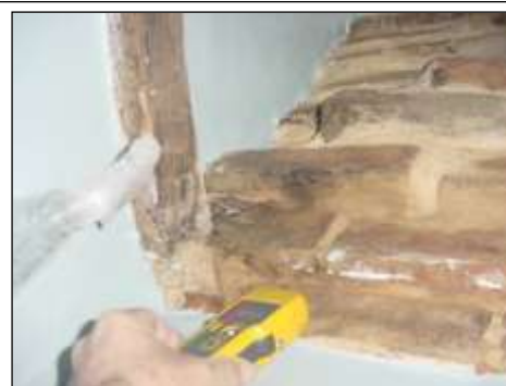
Found a combined dampness problem coming in from the rear left hand chimney (all directions given as you face the property).
