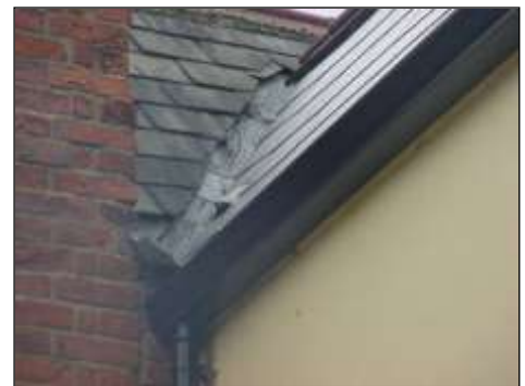
Natural slate to the left hand side and manmade slate to the right hand side and a lead valley gutter that has been tarred indicating that it has leaked
