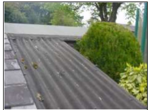
Fibre roof, also to the rear, we would replace with a slate roof in keeping with the rest of the property
