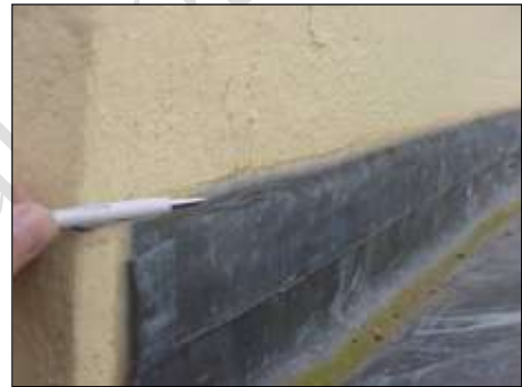
Mastic seal to the lead flashing indicating problems
