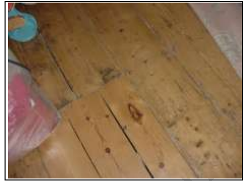
Top Floor: Older timbers have woodworm and there are new replacement timbers
