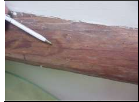
Signs of woodworm in rear building
