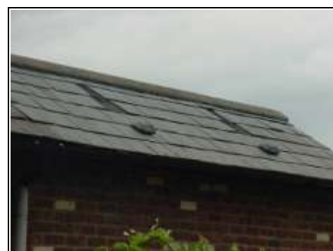
Rear of roof with missing slates
