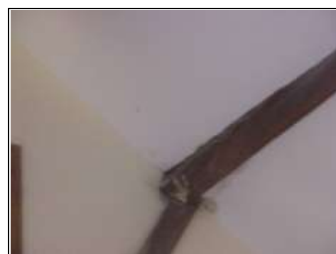
Tingles holding slates in place
