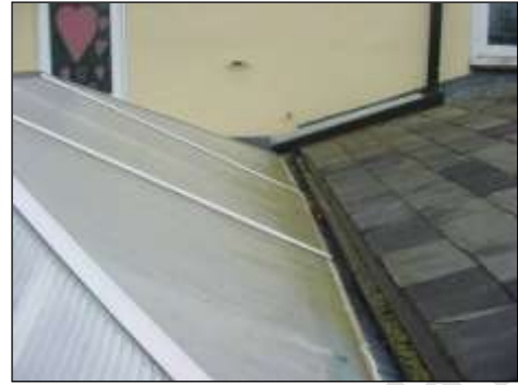
Valley gutter between conservatory and kitchen area
