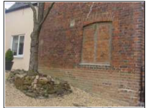
Incorrect cement mortar used to the base of the left hand side of the property for example
