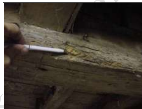
Signs of woodworm in basement
