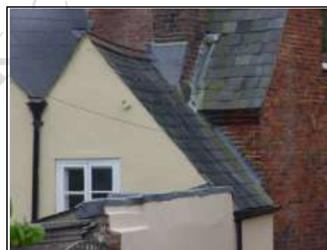
Lead tingles to rear of main roof
