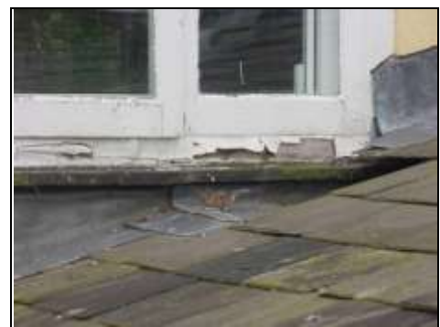
Timber window degrading
