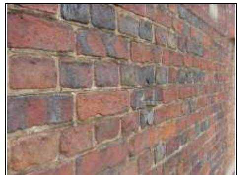
An example of brickwork where the mortar is pinch pointed. If you look closely you can see a line through the mortar.
