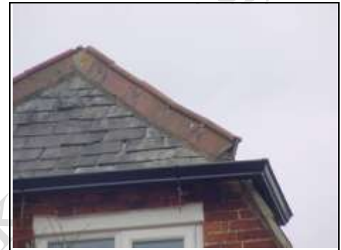
Guttering hiding fascias and soffits
