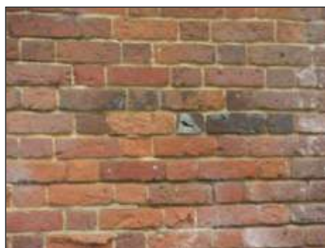
Brickwork in need of re-pointing
