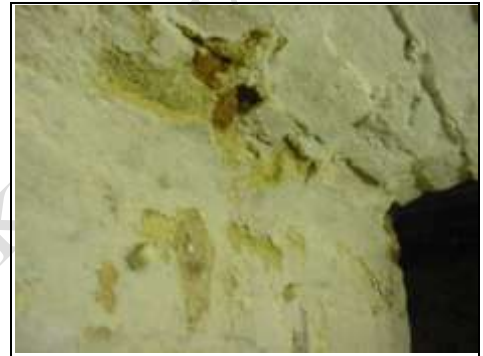
Spalling to chimney
