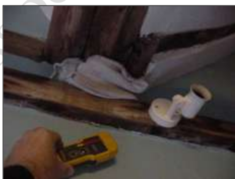
Dampness coming through from the adjacent valley gutter, with cloth in an effort to keep the area dry!
