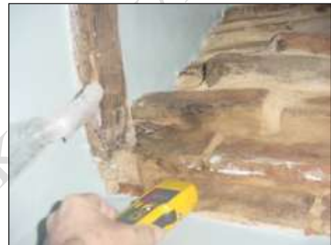
Dampness coming in from chimney one
