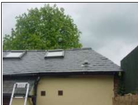
Undulation to rear building roof
