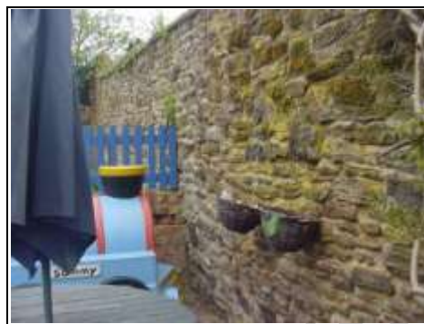
Bulging Boundary wall
