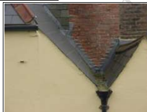
Valley gutter to rear of property at high level
