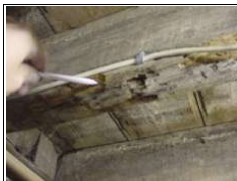
Signs of woodworm in basement
