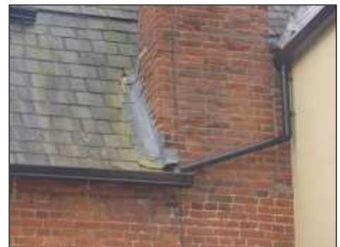
Natural slate to the left hand side and manmade slate to the right hand side and a lead valley gutter that has been tarred indicating that it has leaked
