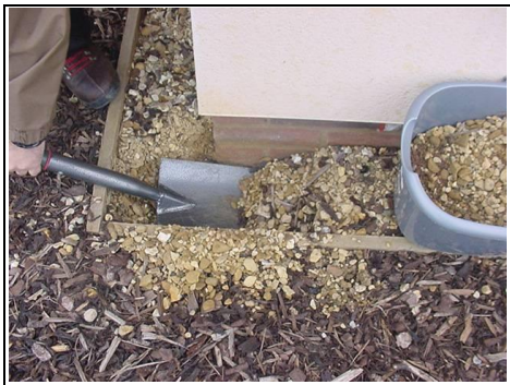
Digging up French drain to front left hand side
