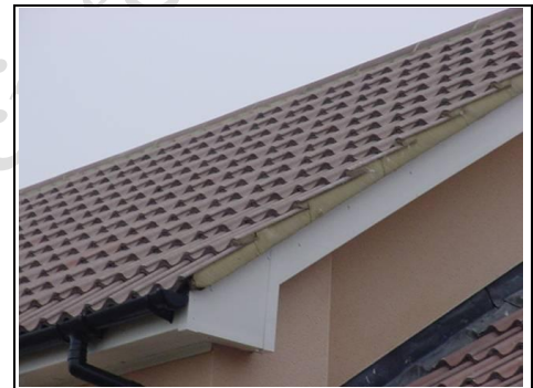
Fascias and soffits
