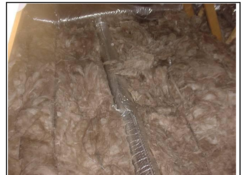
Air vents to roof
