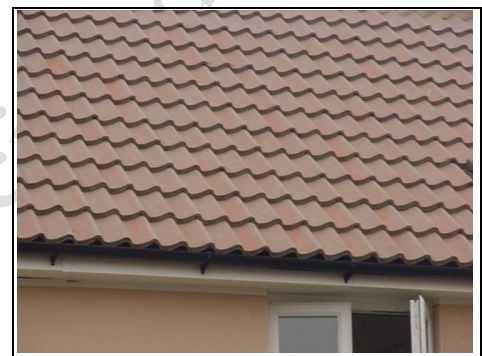
View of the concrete tile roof
