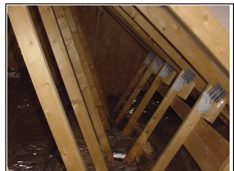
View of roof
