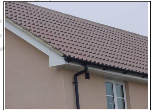
Gutters and downpipes
