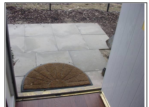
Ground levels have very little difference from outside to inside, a small ramp would have been sufficient to deal with the difference and still allow access to the property under the Building Regulations
