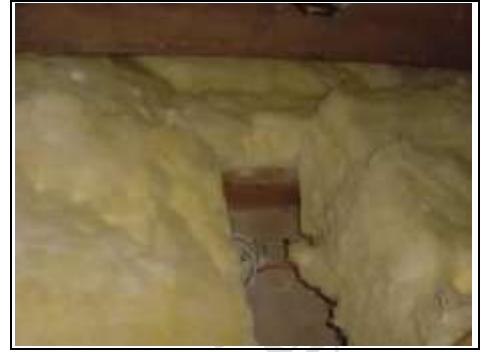
Gaps where lights are is good but shouldn't be covered further
