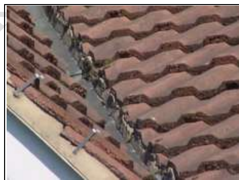
Close up of valley showing the cement is starting to deteriorate
