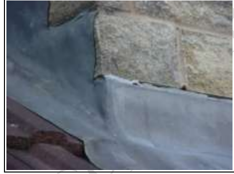
Close up of flashing
