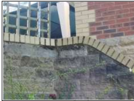
Moss appearing on brickwork and top of stone of retaining wall
