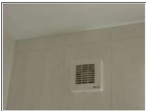
Small extract fan in second floor bathroom
