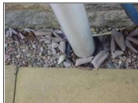
Downpipes going directly into ground
