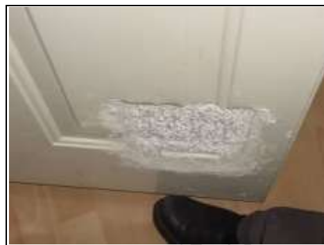
Door to garage damaged. This should be a fire door.
