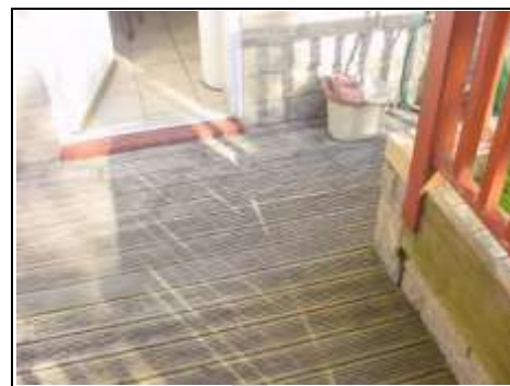
Decking runs directly to the building at rear of property
