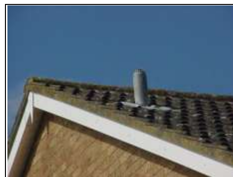
Soil and vent pipe
