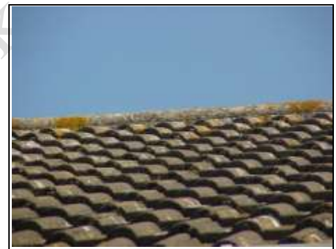
Concrete tiled main roof
