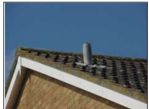
Cement verge looked in reasonable condition
