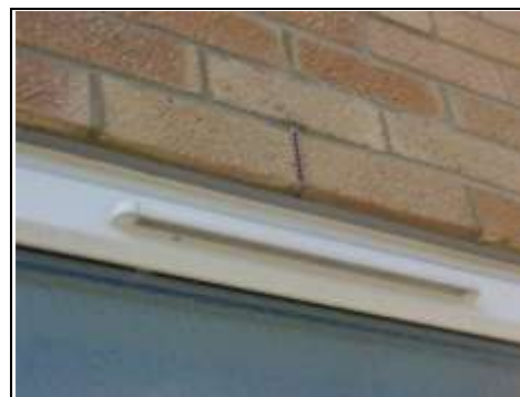
Trickle vents to extension
