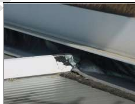
Conservatory roof problem flashing
