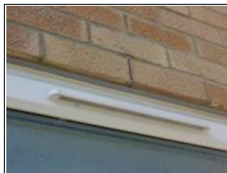
Brickwork with weep hole/trickle vent to the extension
