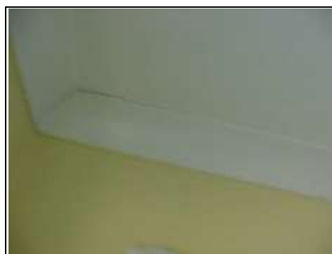
Hairline cracking to ground floor shower room ceiling
