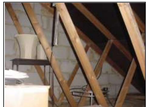
View of roof prefabricated truss
