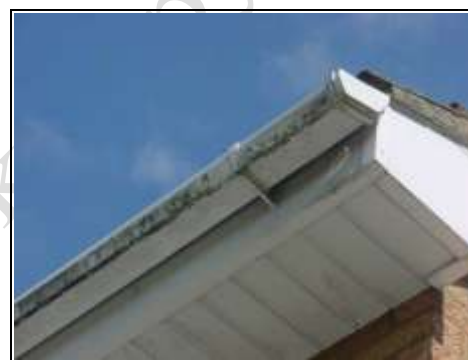
Staining to the rear gutters
