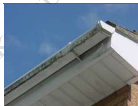
Over clad fascias and soffits
