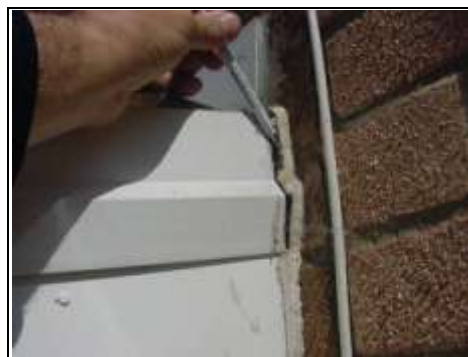
Conservatory roof cover plates coming adrift to the side
