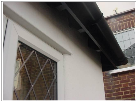
Drip detail over window
