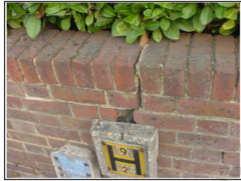
Cracking to boundary wall on left hand side
