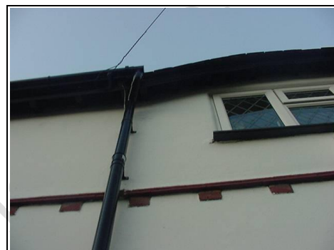
Plastic gutters and downpipes
