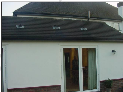
Pitched roof hiding flat roof
