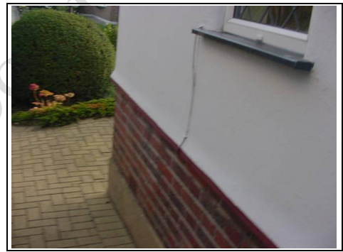
Drip detail to base of the render
