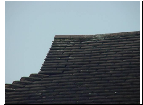
Minor movement to the roof tiles
