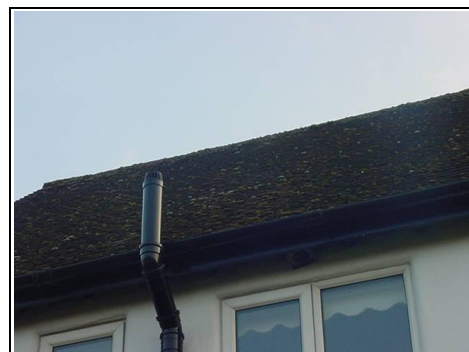
Plastic soil and vent pipe
