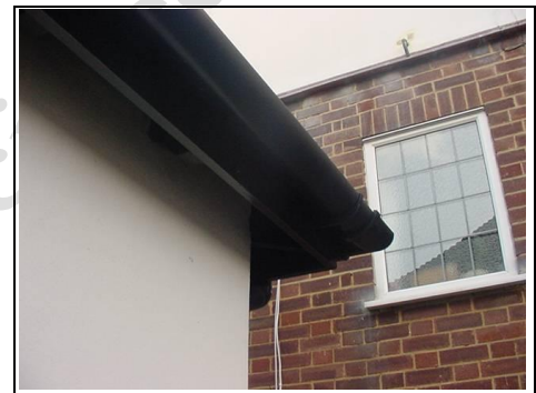
Timber fascia and soffit
