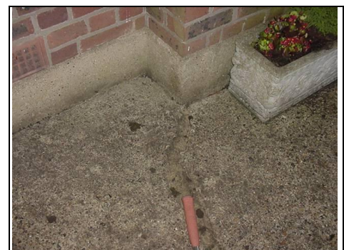
Cracking near to drains
