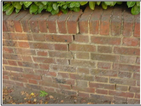
Cracking to boundary wall on left hand side
