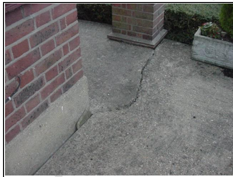
Cracking to rear left hand side
