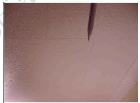
Plasterboard cracks
