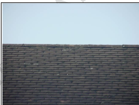
Slight opening up of tiles, hog back ridge needs re-bedding
