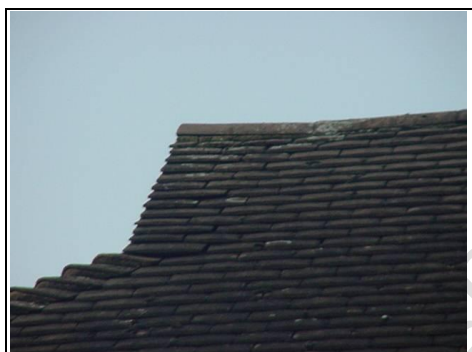
Minor movement to roof tiles
