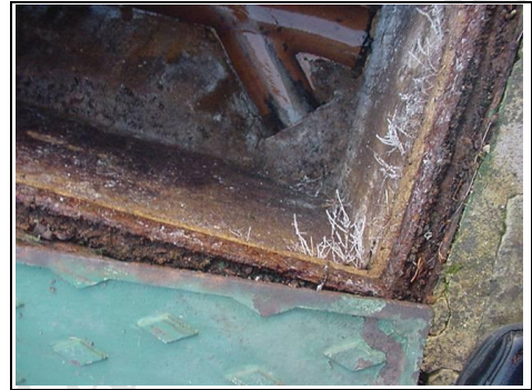
Tree roots in drain
