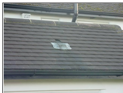
This is the outlet that the water comes from the flat roof
