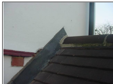
Lead flashing
