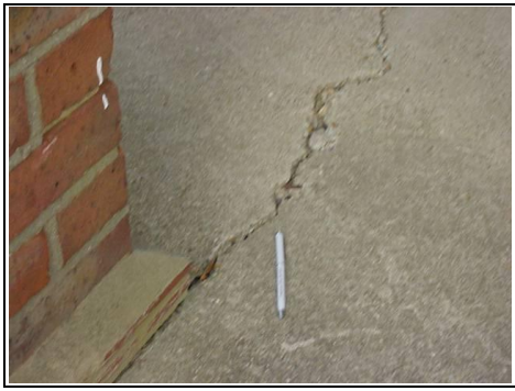
Cracking to left hand side
