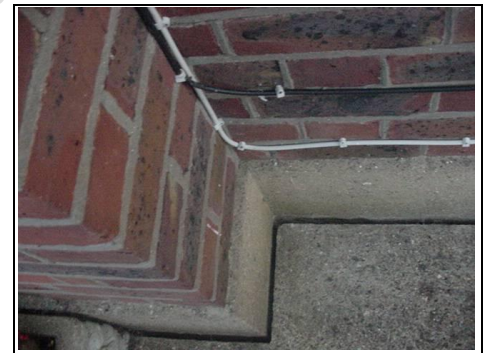
Movement gap between concrete and wall
