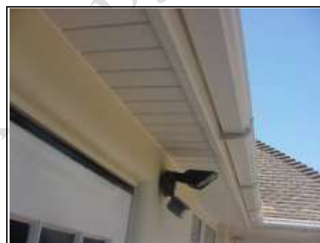
Fascias and Soffits are over clad
