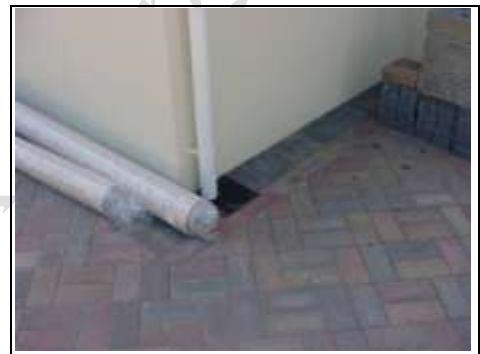
Lack of Bell Mouth Detail to base of Render
