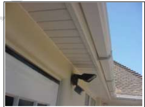
Over cladding on Fascia and soffits
