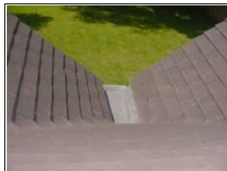
Valley Gutter to the Rear. We think that this will block in years to come as it is a poor detail.
