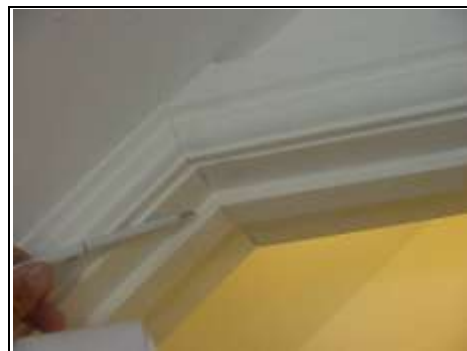
Opening up of architraves around the doors
