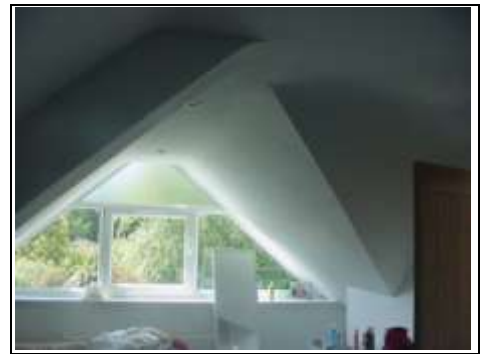
Drop beam infringing on ceiling and room height
