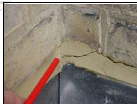
Cement mortar has been used to point in the lead flashing. We much prefer mastic as it's longer lasting
