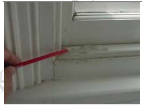
Dampness coming in through bathroom window. This may be due to condensation but may be due to leaking gutters
