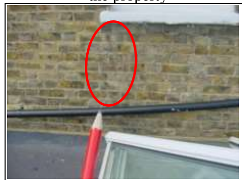
Hairline cracking
