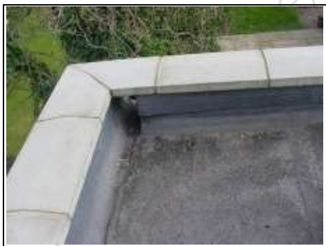
Some pattern staining on the roof indicating water is ponding on the roof.
