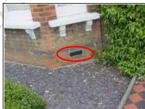
Air brick to front bay window area with air flow underneath
