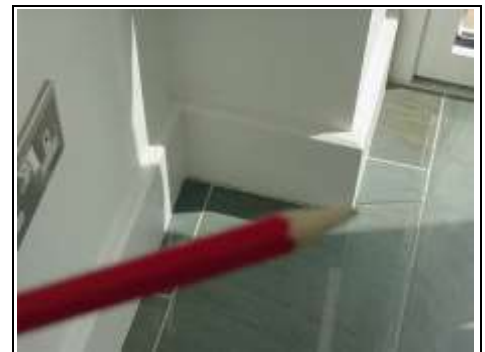
Tiles cracked in kitchen because no expansion joint around the tiles
