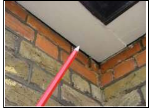
Soffit board a fraction away from the building. Is this intentional for the room in the roof or due to movement?
