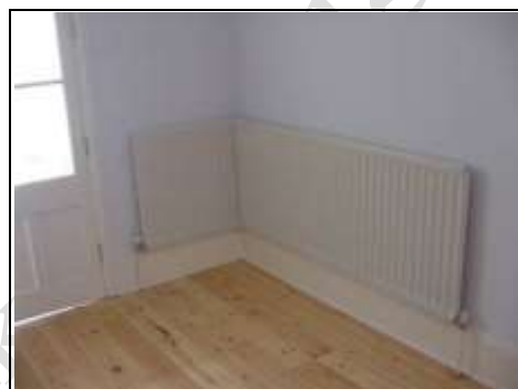
Internal single panel radiator
