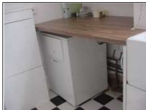
Floor mounted Worcester boiler
