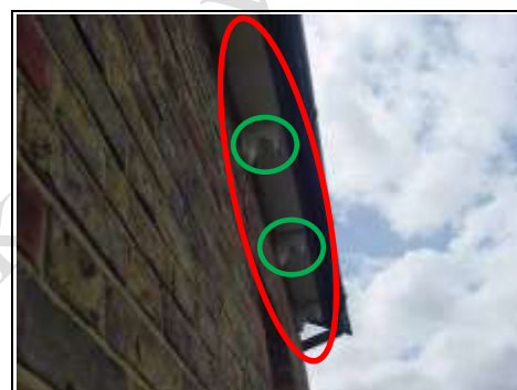
Fascia and soffit (red oval) Corbels (green circles)
