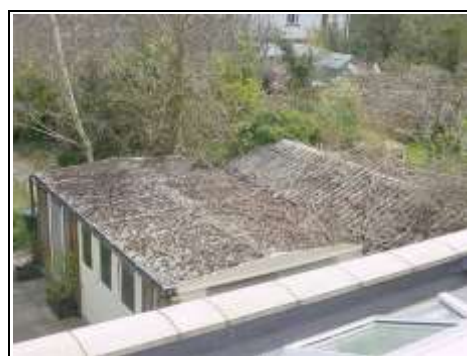
Asbestos roof on garage
