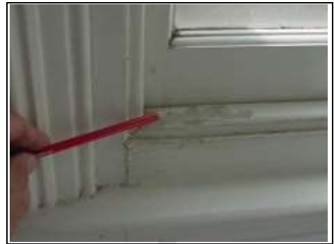
Dampness to bathroom window
