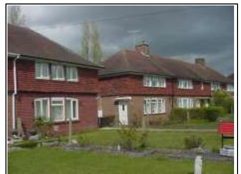
Post war 1960's properties with plastic double glazing without trickle vents that have been added can cause condensation.
