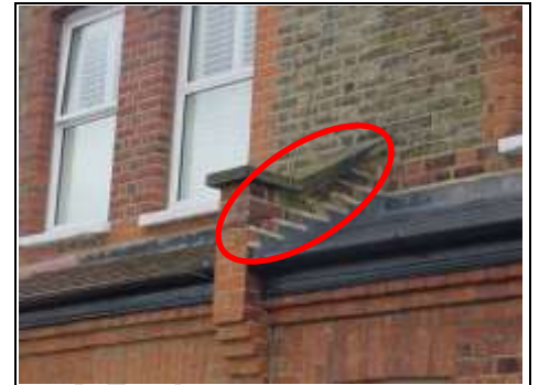
Parapet wall re-pointed in cement mortar. Just a reminder that you may have to re-point this
