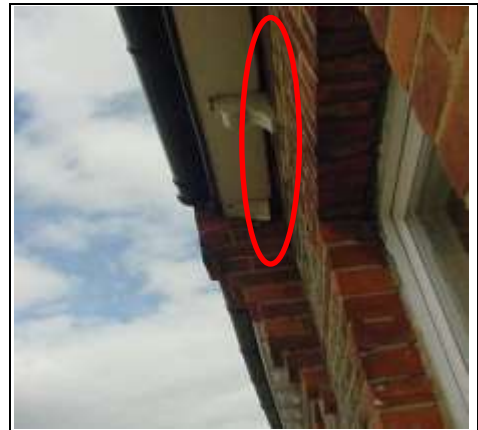
There is a gap between the wall and the soffit.
