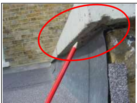
The coping stone does not have a sufficient drip
