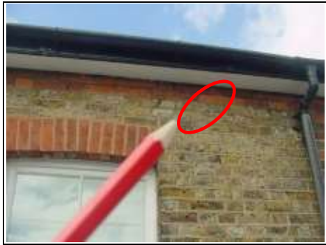
Cracking to the rear of the property
