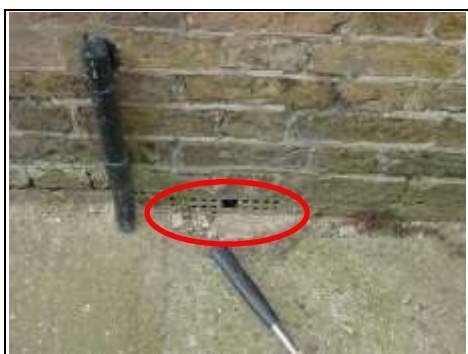
Partly blocked air brick on this property (right)
