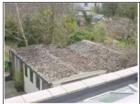
Asbestos roof on garage
