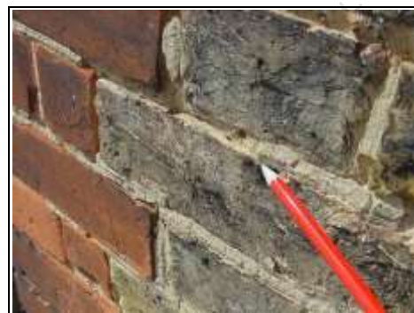
Re-pointed in cement mortar instead of lime
