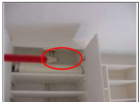
Cracking to the rear bedroom in the cupboard
