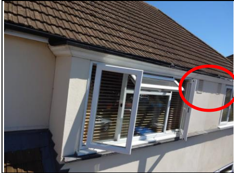
High level airbrick to the front Ariel view – 360 photo
