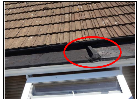
Split in the felt to the front flat roof Ariel view – 360 photo
