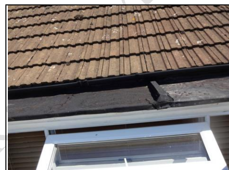
Split in the felt to the front flat roof above the boxed bay window
