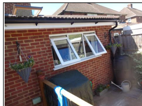
Plastic double glazed windows with trickle vents Ariel view – 360 photo
