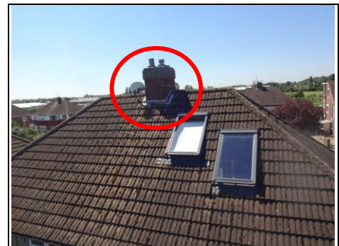
The flashing to the chimney needs to be checked Ariel view – 360 photo
