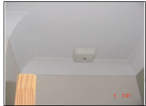
Battery fire alarm
