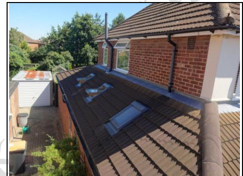
Stretcher bond brickwork
