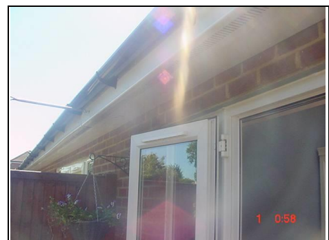
Plastic double glazed door with trickle vent
