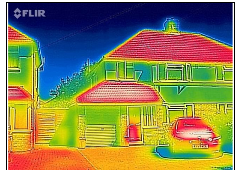
Thermal photo Showing the warm roof in red
