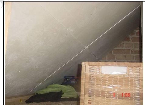
The underside of the roof which was lined with plasterboard
