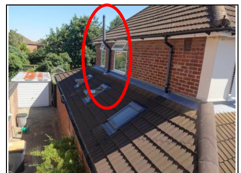
Soil and vent pipe Ariel view – 360 photo
