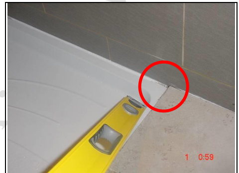
Black mould in the internal shower room
