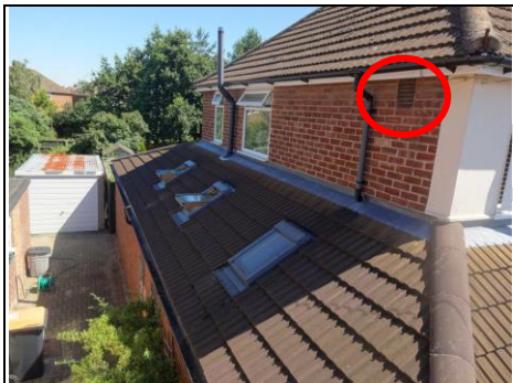
High level airbrick to the left side Ariel view – 360 photo
