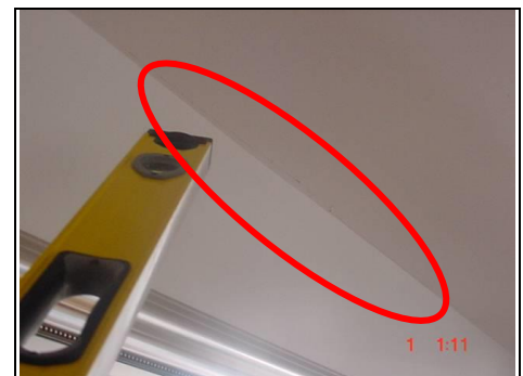
Hair line cracking to the rear reception room
