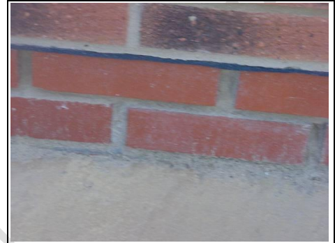
Unusual detail as no mortar in some of the joints
