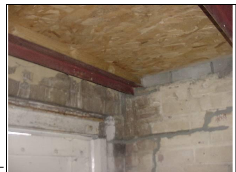
Metal joists in garage roof
