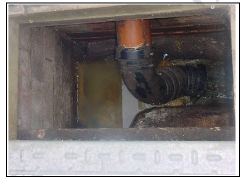
Internal manhole not to building regulations
