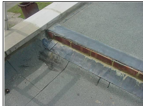
Poor detail to parapet wall
