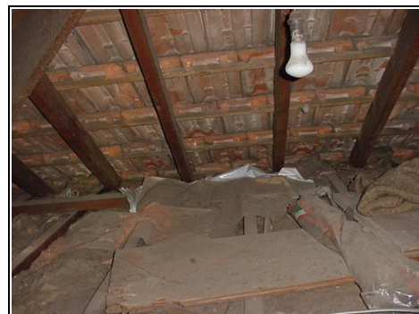
Lack of roof insulation
