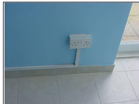
Surface mounted electric wiring
