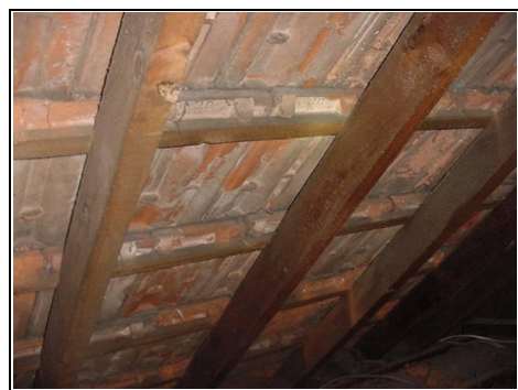
No felt in roof
