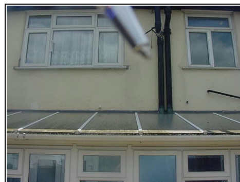
Cracks to render
