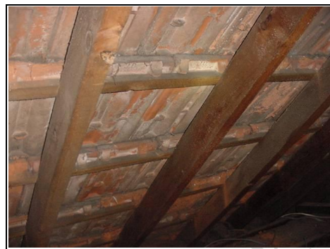
No underfelt in roof
