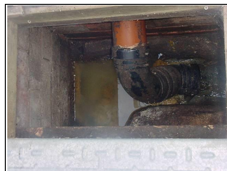
Internal manhole – not to building regulations
