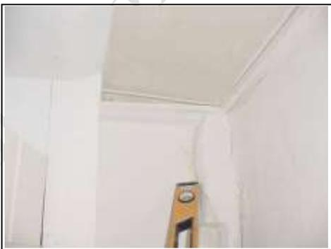
Wall to ceiling crack in the link corridor, first floor
