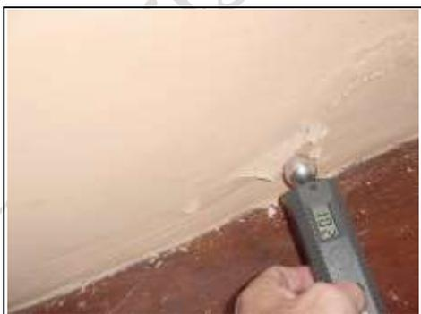
High dampness level noted under the window in the hallway
