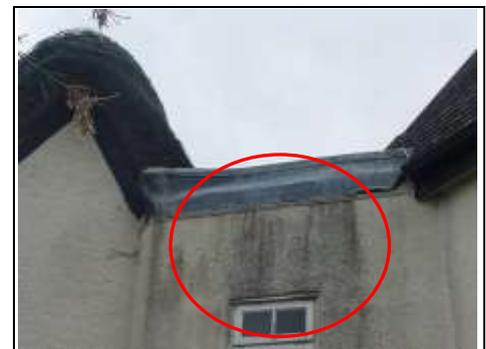
Pattern staining to the rear of the property due to the lack of detail
