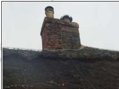
Rear of the chimney has a crack between the two chimneys
