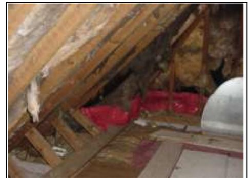
Cut timber roof with props added, often after roof spread
