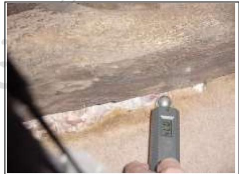
High reading of 74 to the stone/tile below the sole plate explains the rot
