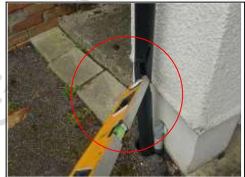
Damage visible to the downpipe left of the garage door
