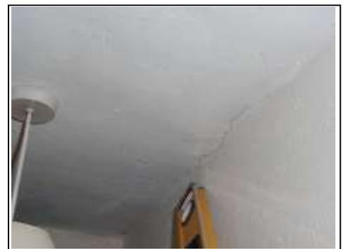
Cracking where the old building meets the new
