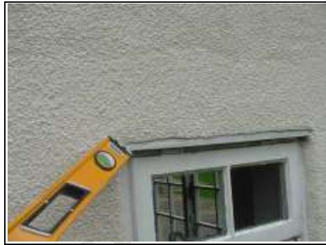
The original drip in the wood has been lost due to the render
