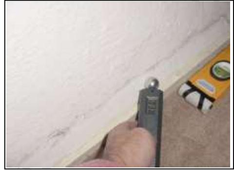
Damp readings taken where the sole plate should be – slightly high
