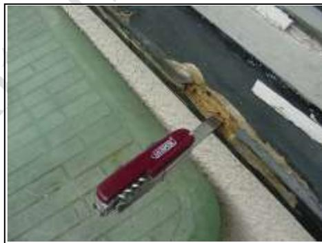
Knife test in window – timber has deteriorated
