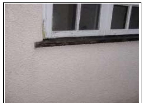
There was no obvious crack noted on the outside of the wall in relation to the damp under the window
